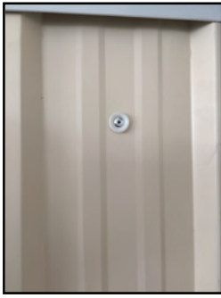
rivets with washer
